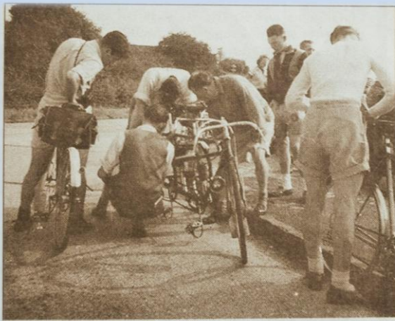
Repairs-Trouble with a tandem
